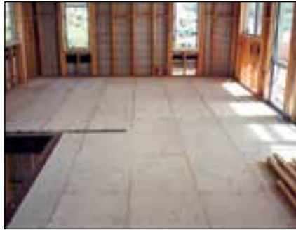
Fig 1.1.2 Residential Suspended First Floors
