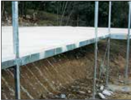
Fig 1.1.1 Residential Suspended Ground Floors
